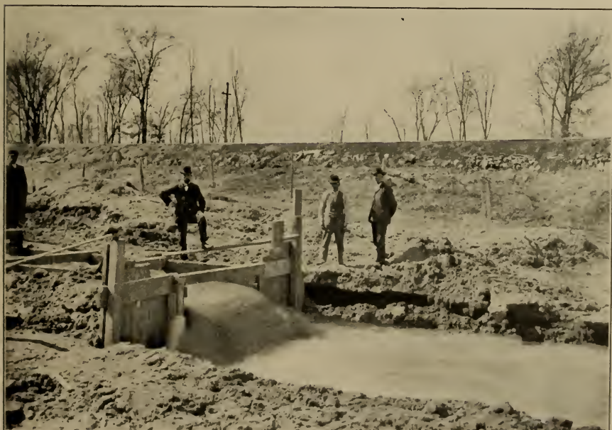
WEIRING THE WATER—MEREDOCIA DRAINAGE DISTRICT. 25,000 GALLONS PER MINUTE.
